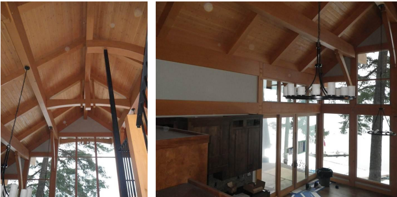
Fig.3.17 Cathedral ceiling and timber frame construction viewed from the inside of test house #3, Chase, BC.
