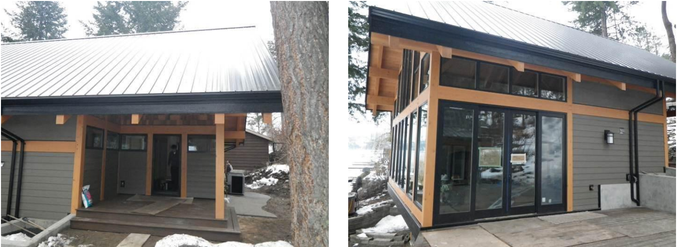
Fig.3.16 Air-tightness test house #3, Chase, BC.
